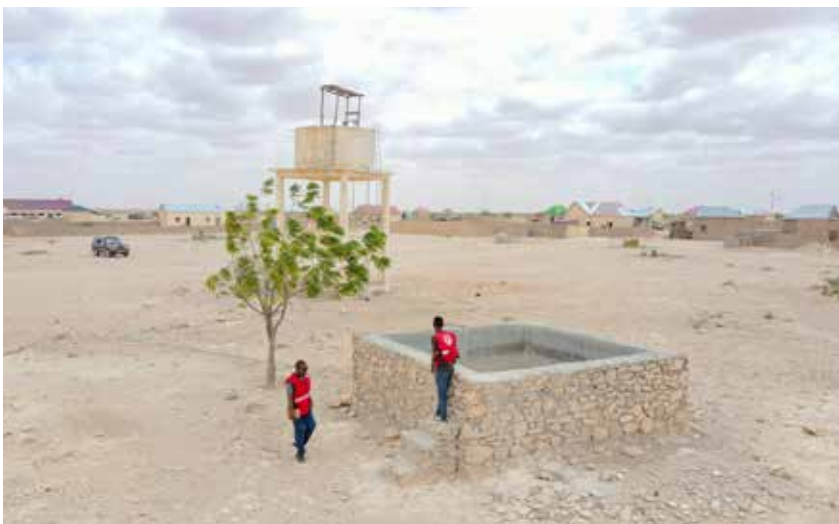
Gacnafale village in Somalia has many water wells, but the taps are dry. "We need fuel and diesel to run the pumps," says the village chief. "The situation here is not good at all because we have limited resources and now we have to buy water."
